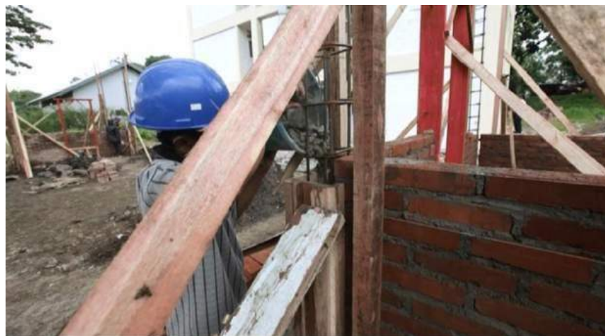
Gambar II.415 Proses Pengecoran Kolom
