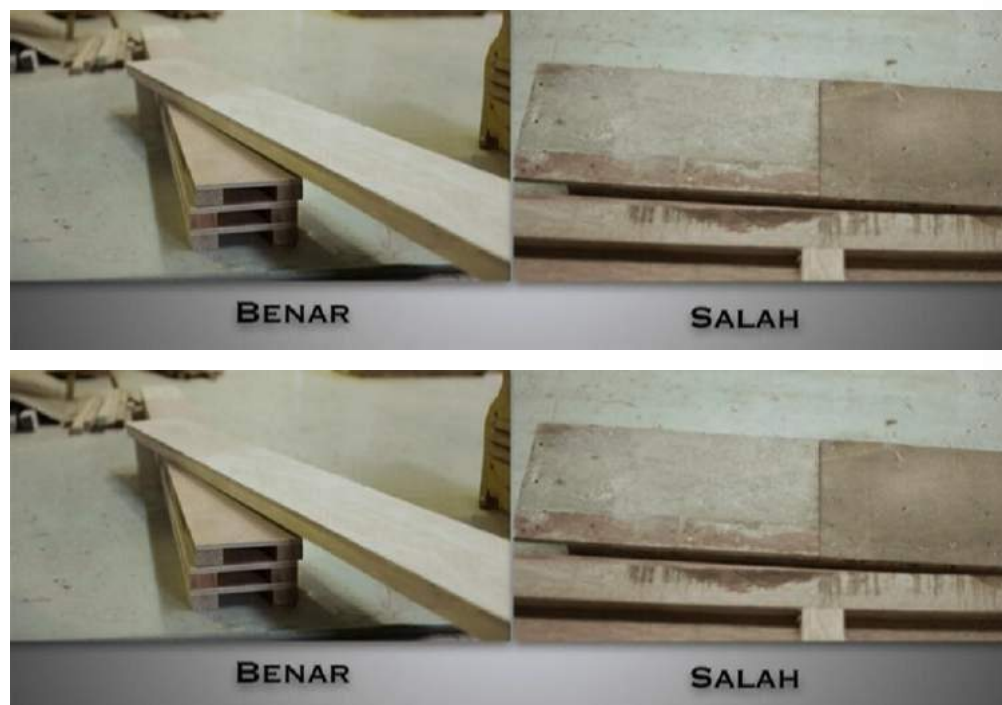
Gambar II.413 Kualitas Cetakan/ Bekisting
