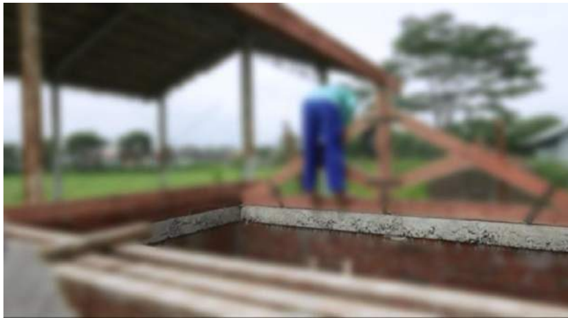
Gambar II.381 Balok Keliling/ Ring
